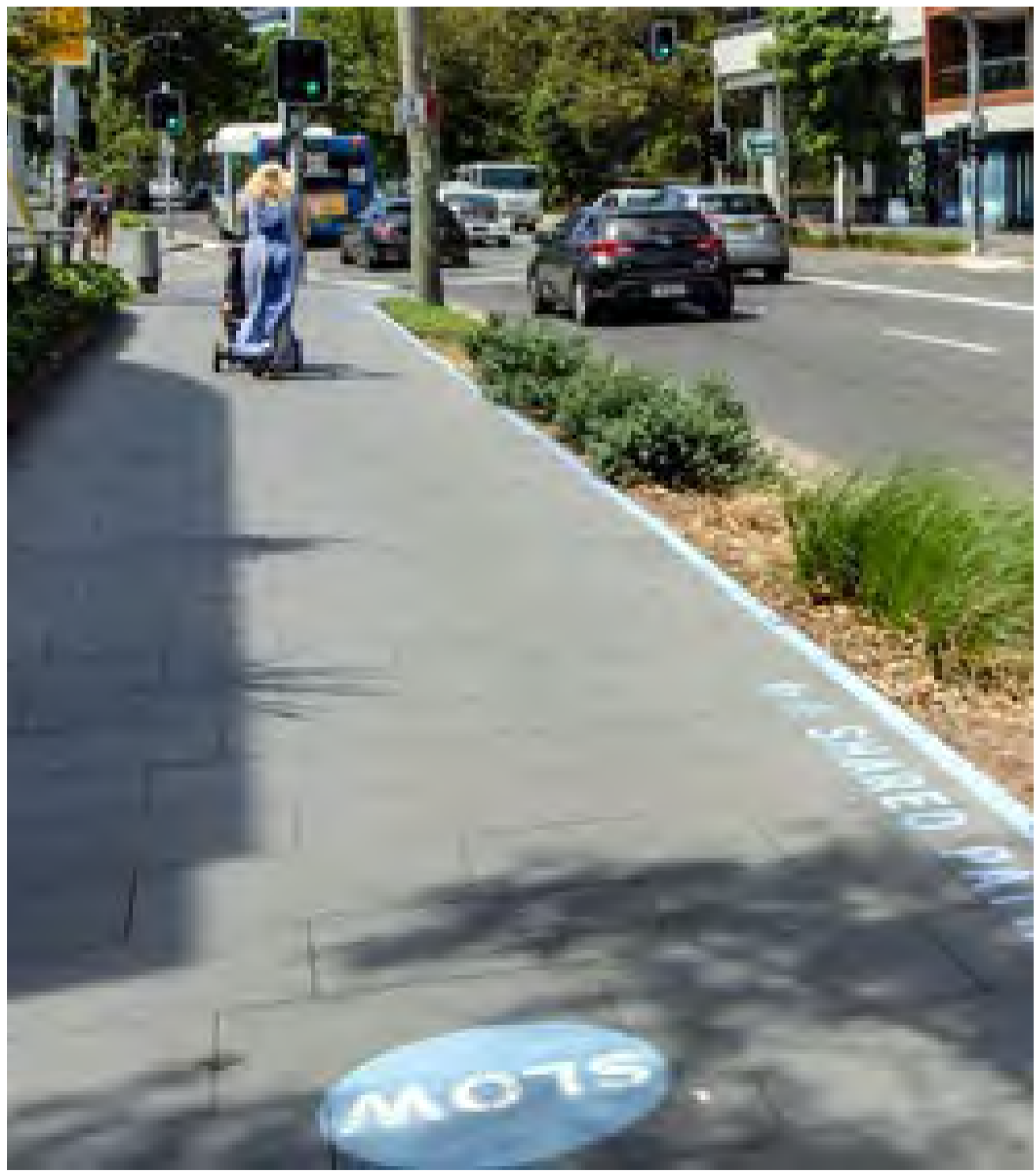
FOOTPATH UPGRADE & WIDENING FOR INCLUSIVE USE
