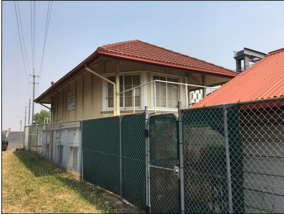
Figure 15: Lidcombe Signal Box viewed from Railway Street.
