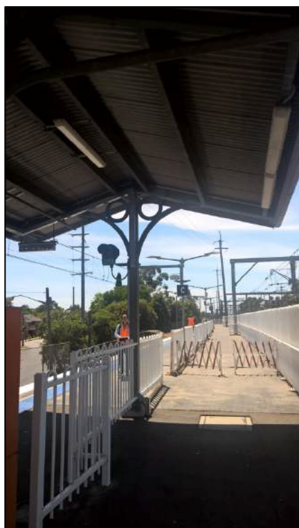
Figure 11: Platform 0, looking east towards the subject site.
