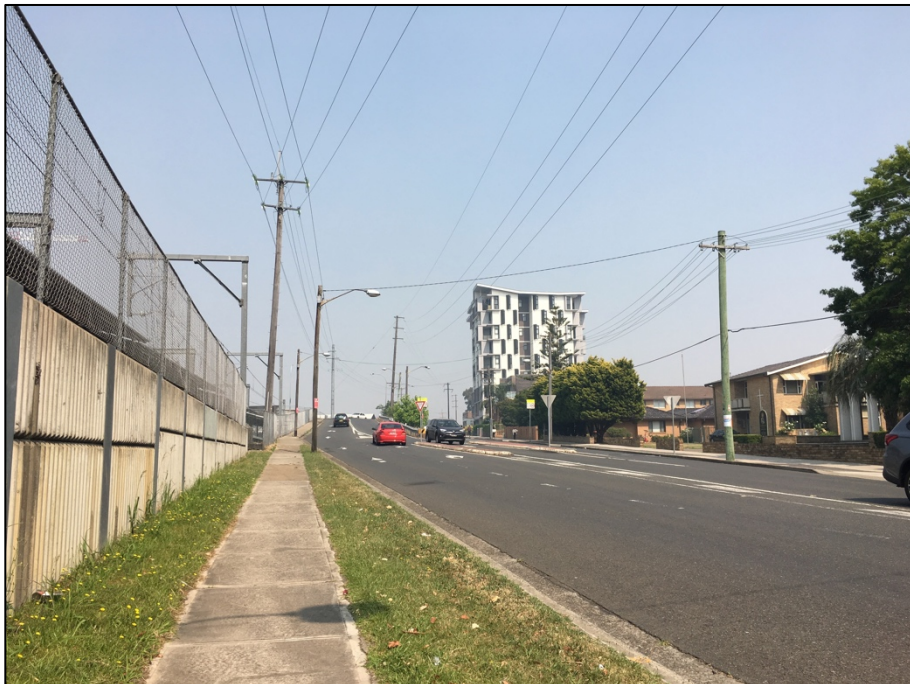
Figure 13: View west from station towards Lidcombe town centre along Church Street.
