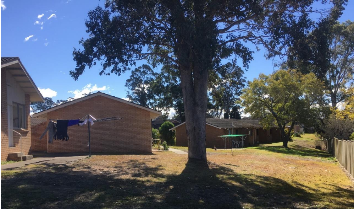
Figure 3: Typical single storey independent living units adjacent to the eastern boundary
