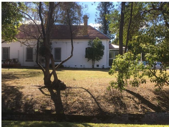
Figure 12 Sherwood Scrubs building to the west
