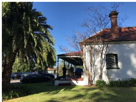
Figure 23: North east corner of the house, showing a side-view of its front verandah (Source: NBR
