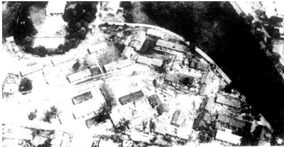
Figure 8: 1973 photograph showing the nearly completed Stage 1 of the Cardinal Gilroy Village. Cerdon House, originally known as 'Sherwood Scrubs' and later part of Cerdon College, is visible at the top left. (Source: People enter village, The Broadcaster , 6 March 1973, p1)
