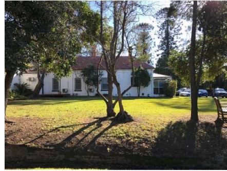
Figure 26: Southern façade of the house, viewed from the channel adjacent to the boundary to Cardinal Gilroy Village (Source: NBR SARCHITECTURE)
