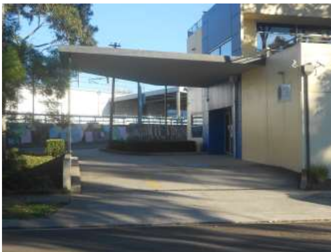
Figure 5 – Main entrance to the existing building (from Percy St)
