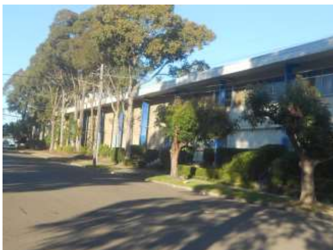
Figure 4 - View of the existing building from Percy Street
