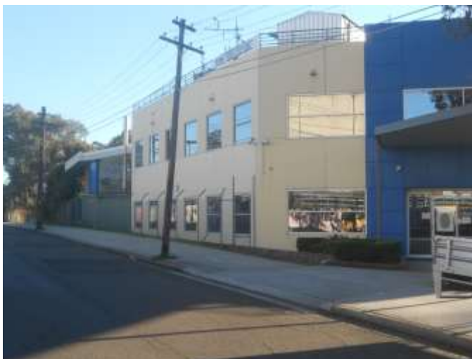
Figure 6 – Existing two storey administration building located along Gelibolu Parade
