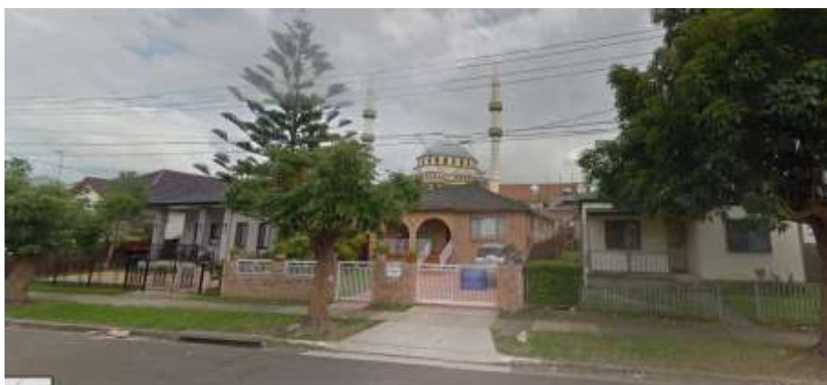
Figure 9 - Views from St Hillers Road showing the existing low density residential area
