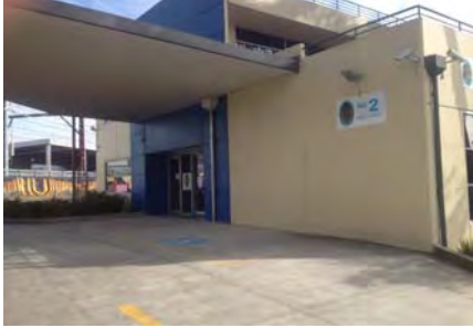
View of: Office building and site entrance Looking west Inspected on 23.04.14
