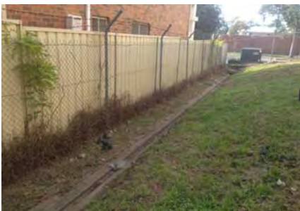
View of: Stormwater drainage line Looking east Inspected on 23.04.14
