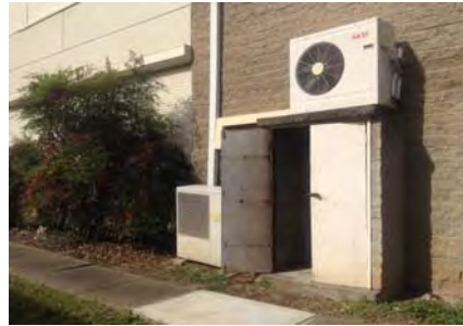
View of: Back entry of the warehouse Looking southeast Inspected on 23.04.14
