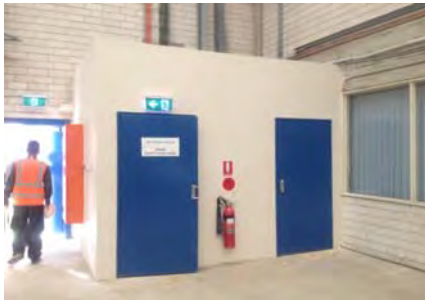
View of: Substation area Looking north Inspected on 23.04.14
