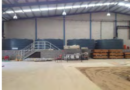
View of: 4 large detention tanks Looking north Inspected on 23.04.14
