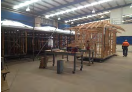
View of: Training area Looking west Inspected on 23.04.14
