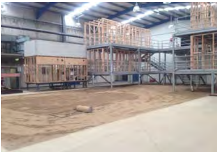
View of: Sand pit area inside warehouse Looking east Inspected on 23.04.14
