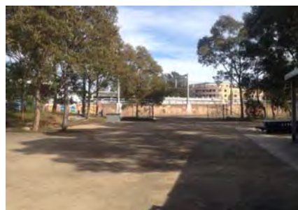
View of: Car park area Looking west Inspected on 23.04.14
