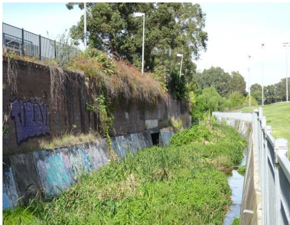
Channelised section of A'Becketts Creek
