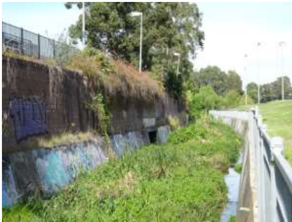
Channelised section of A'Becketts Creek
