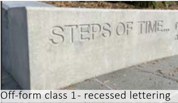
Wall top edge - polished finish or off-form class 1
