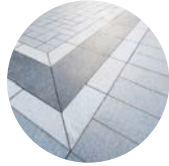
Decorative paving with artworks for areas of social gatherings including playgrounds and outdoor dining areas.
