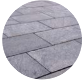
New pebblecrete pavers within the local centres
