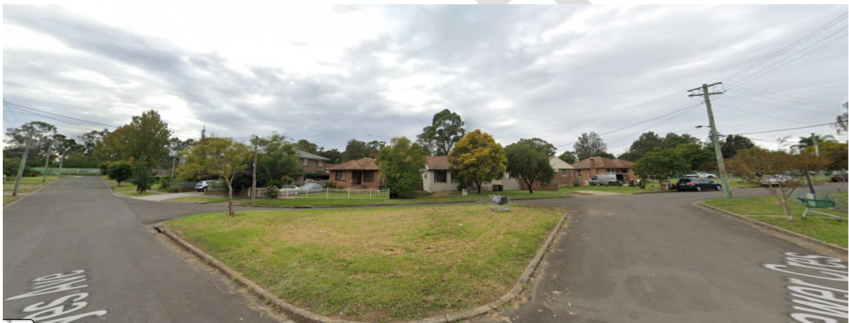
Figure 4.32: View of looking north at the intersection of Brewers Crescent and Hayes Avenue South Wentworthville showing existing low density residential character. Source: Google Streetview, accessed 2024.
