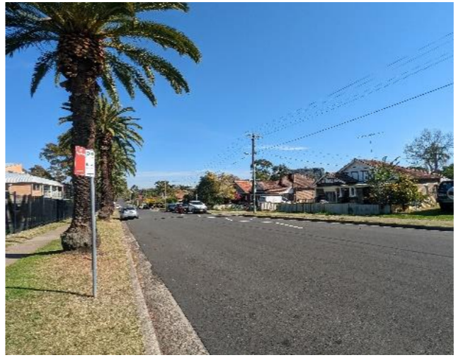
Looking north west along Moree Avenue, with public school to the left and HCA to the right.
