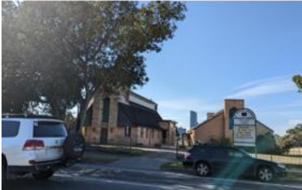
Figure 7.4 View of St Barnabas Anglican Church from opposite side of Hawkesbury Road.
