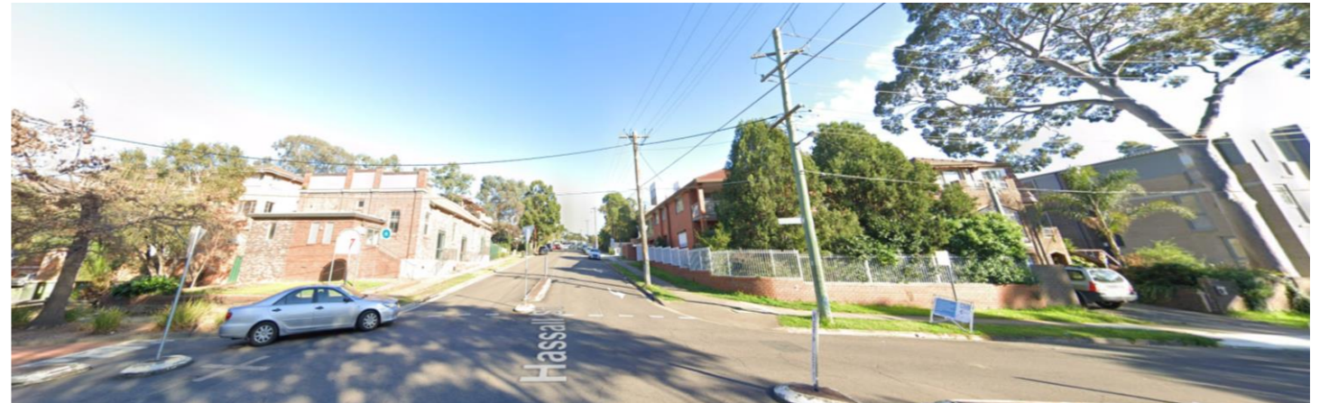
Looking west along Priddle Street, with Westmead Progress Hall (I279) to the left. The Buildings to the right will potentially be up to 12 storeys high.
