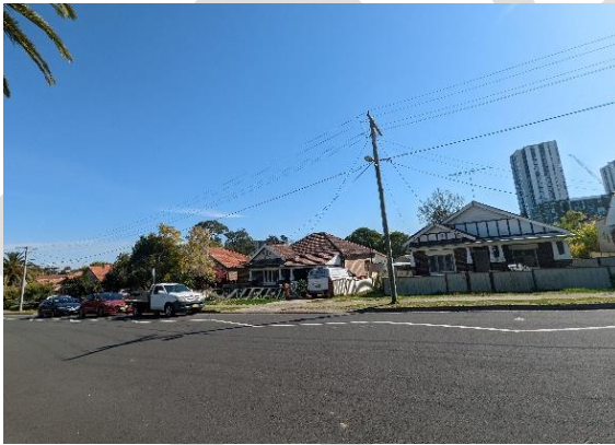
Figure 7.7 View looking north towards Heritage items within Toohey's Estate HCA fronting Moree Avenue,
