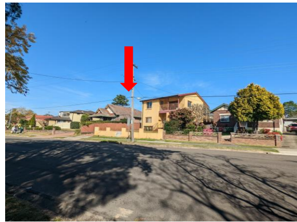
Looking south down Houison Street, showing the proposed heritage item, 74 Houison Street (identified by red arrow). Up to eight storeys proposed for residential apartments immediately adjacent.
