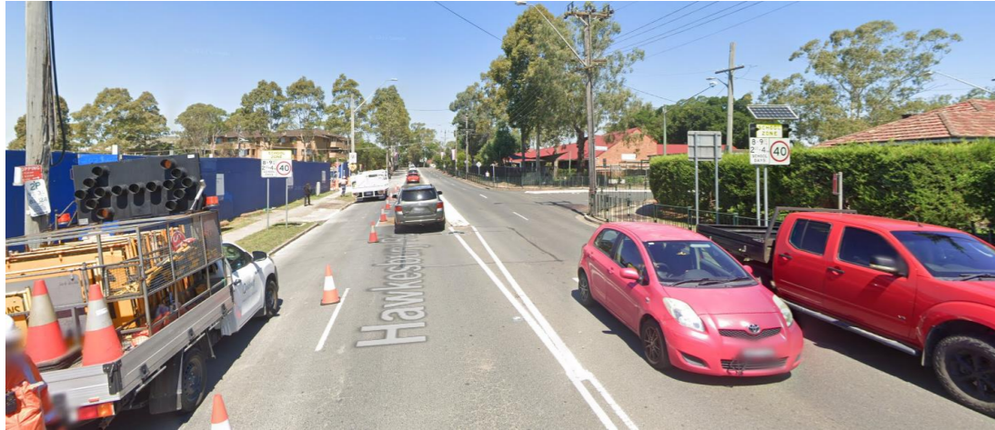
View south down Hawkesbury Road towards Westmead Public School and existing residential development. New Metro Station construction hoarding (left). Up to 20-25 storeys high residential scale proposed for residential blocks within this vicinity.
