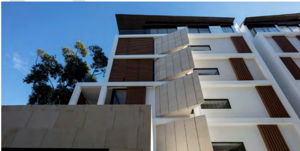
Figure 12. Example of building providing visual screening including 'wing windows' to minimise overlooking across side boundaries
