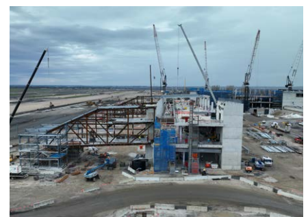
WSI terminal construction
