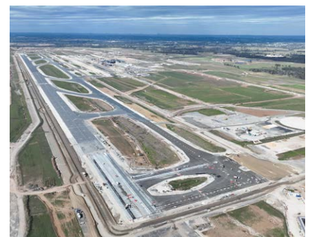
WSI runway construction
