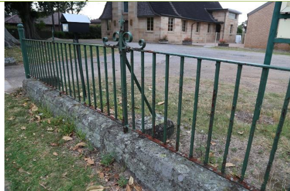
Wrought iron fence on sandstone base.
