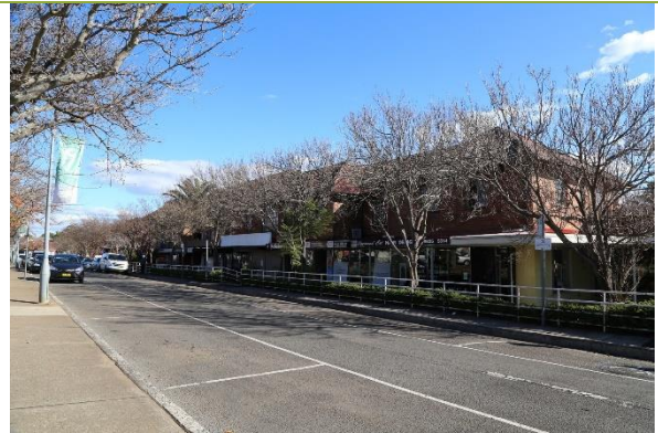
Overview of building.
