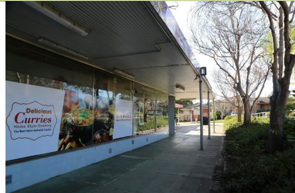
Detail of shopfront at the northern end of the building.
