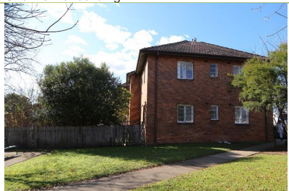
South elevation of building.
