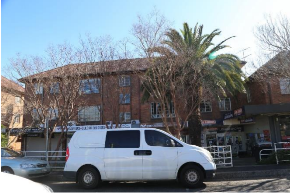
View from parking bay to front façade.
