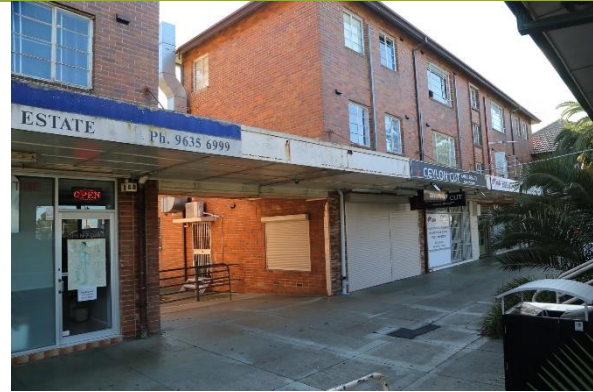
Middle of buildings, adjoined by awning.
