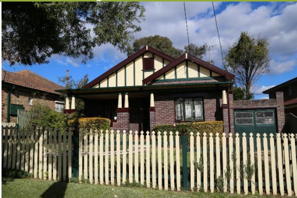
Front façade as viewed from Austral Avenue.
