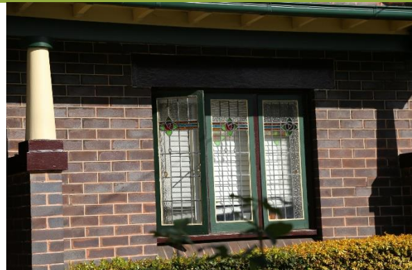
Detail of leadlight casement windows.
