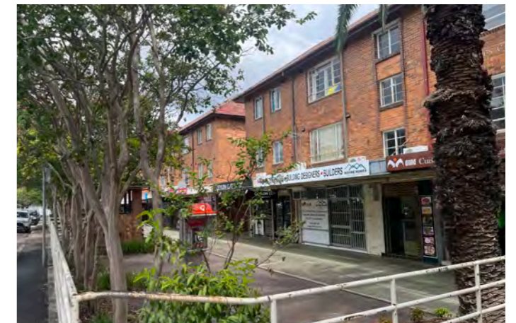
View towards existing shop top housing within the Oakes Centre
