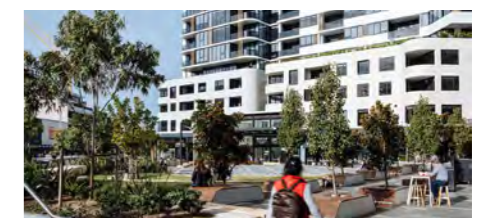
Apartments overlooking public plaza (Lighthouse, Dee Why)
