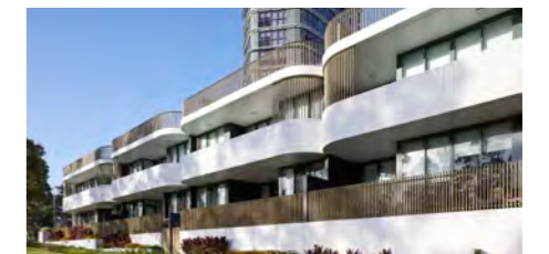
Fine grain podium/street wall with towers well setback (Carter Street, Olympic Park)
