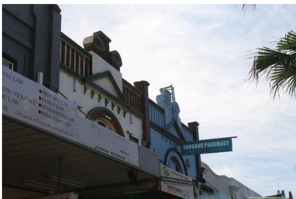
View from footpath to 23-25 Auburn Road.
