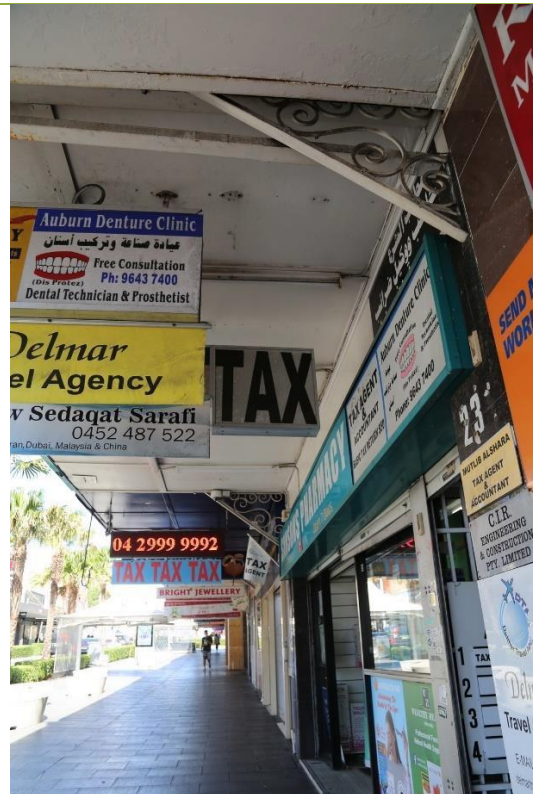
Underside of awning.
