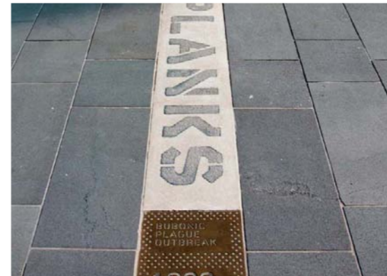
TEXT INLAYS IN CONCRETE PAVING BANDS (site specific narrative text embedded)
