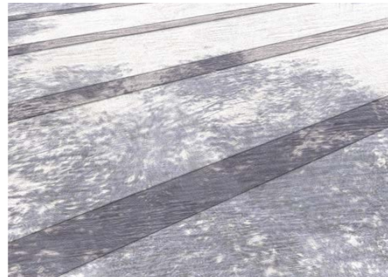
PEBBLECRETE PAVING BANDS
